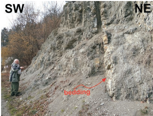
Fig. 6. The Czerwoniak Mt., roadcut exposure at Krosnowice. Photograph shows vertical Turonian calcareous mudstones. Photo taken by M. Rauch, J. Badura as a scale.
